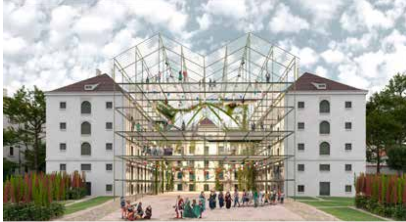
AKVS got a Special Mention in E16 for their project „Medieval Experimentarium“. It infuses life into the historical milieu of the old prison building of Landshut. A light steel structure, a skeletal double of the two prison wings, is inserted into its courtyard to act as a support system
